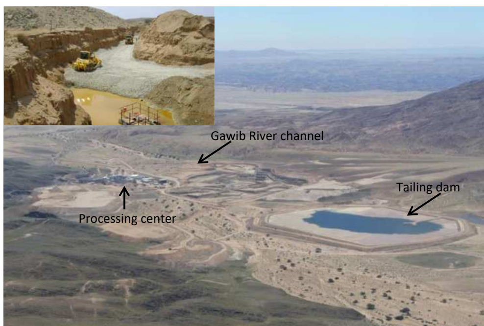
Figure 2. Uranium mine tailing at the Langerheinrich mine overlying the Gawib River channel with an inset showing seepage from the mining operations.
