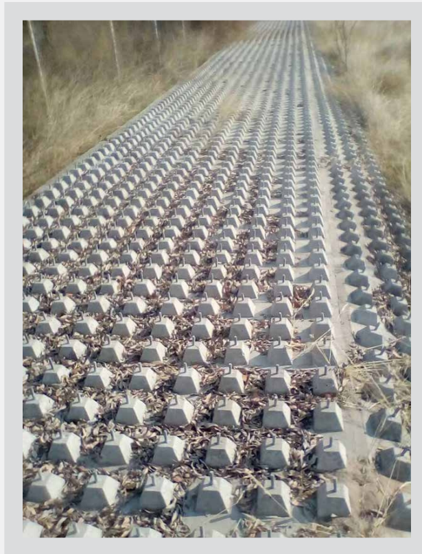
Figure 6 Concrete and steel device to prevent elephant access (Source: photo distributed on social media without copyright)
