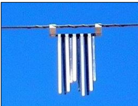
Lithops-Walmund: Swakop River to Walmund, showing two types of mitigation devices fitted onto the new line 12/11/14
