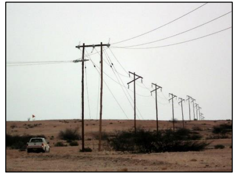
Rössing Uranium: X-mas tree structure (left) and A-frame (centre; 30/7/14); wishbone structure (20/8/14)
