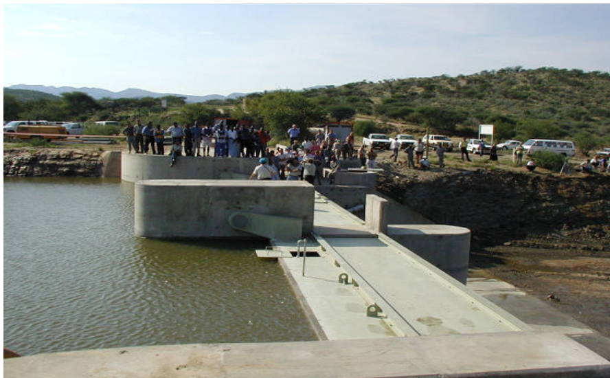
Gates ready for wet commissioning
