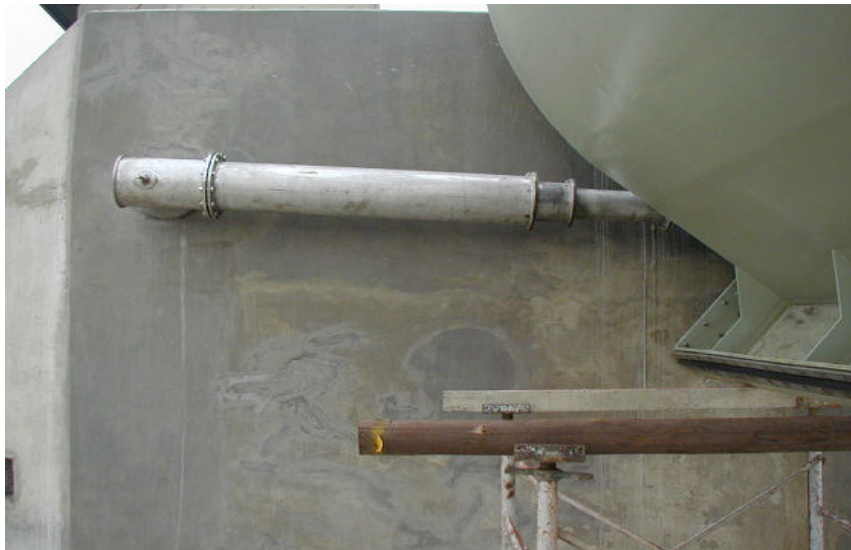
Telescopic arm connecting the ballast tank to the float controlled valve.
