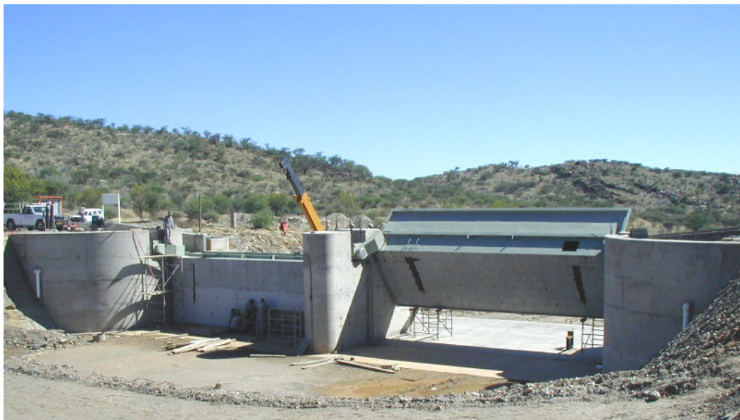
Gates installed ,one partially open
