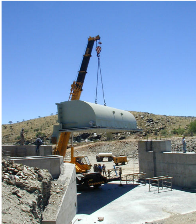
Gate lifted complete into position
