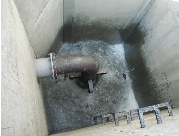
Float controlled discharge valve discharging water from the ballast tank
