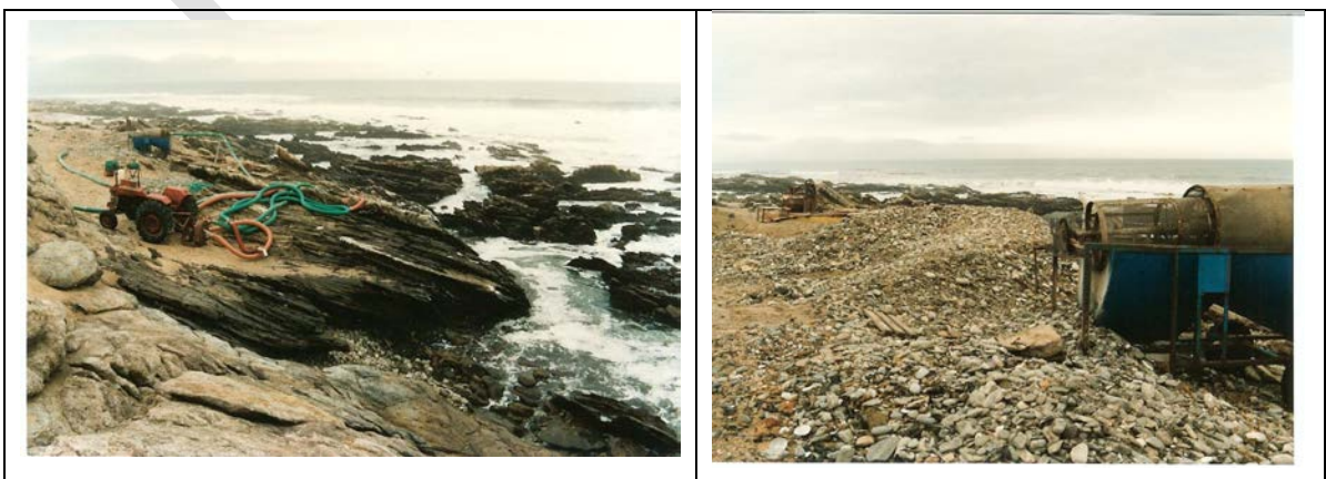
Plate 5.5: a) Tractor and suction hoses; b) Mounds of oversize stones next to the classifier
