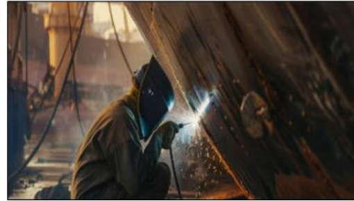
Figure 4: The typical welding process
