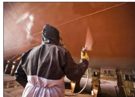
Figure 6: The typical steel hull painting process
