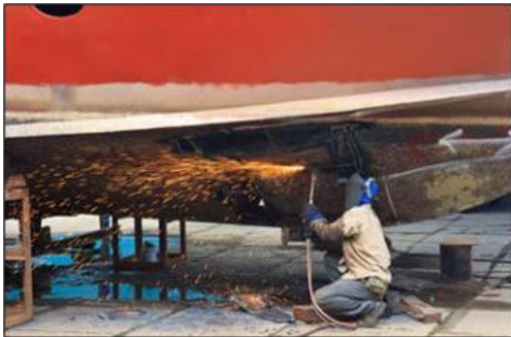
Figure 2: A typical image of cutting with a flame torch
