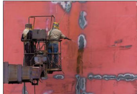
Figure 5: The typical grit blasting process
