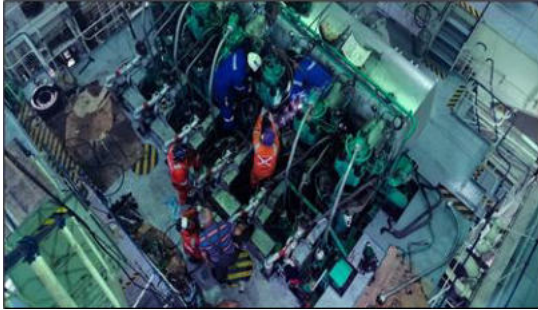
Figure 8: Main Engine overhaul works
