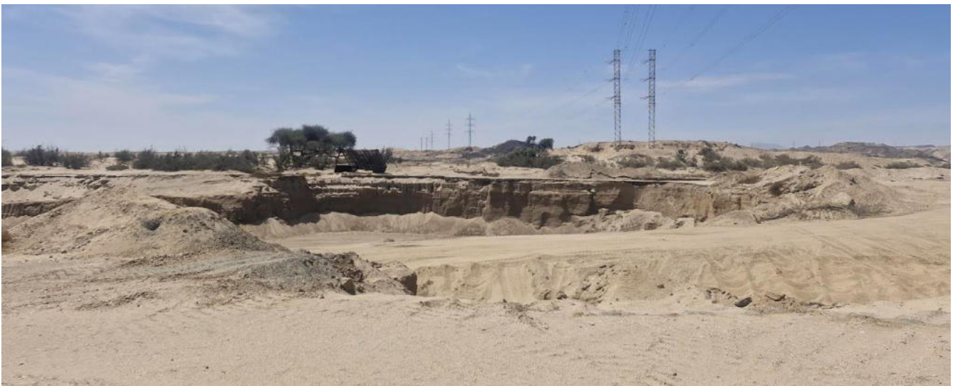
Figure 3: Sand mining pit at current site
