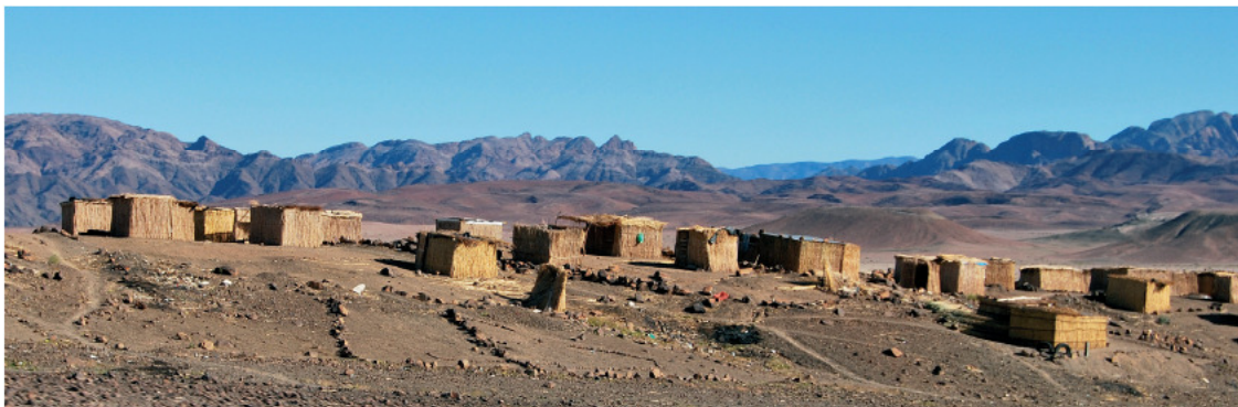
This housing along the Orange River is constructed using locally available reeds.
