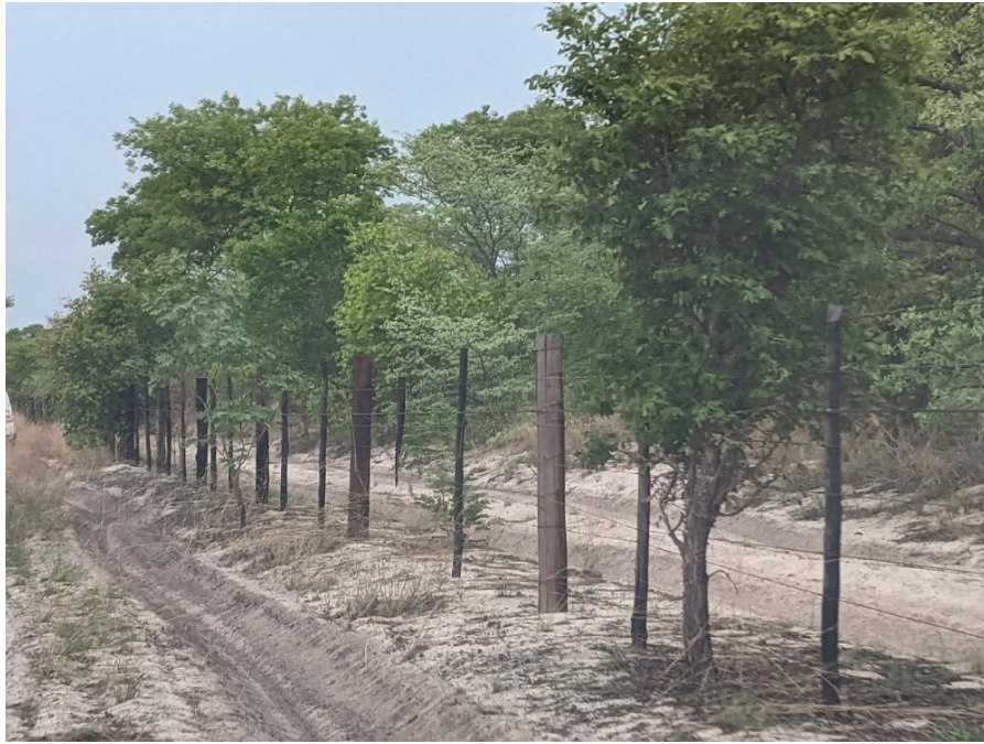
Figure 17. Northern Buffalo fence in good condition, although with a lack of bush-clearing, as observed during a site visit in November 2022.
