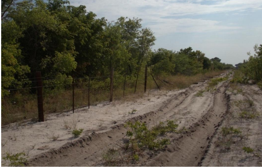
Figure 12. Eastern Zambezi Border fence, showing intact and upright fence posts followed by a section of downed posts and wires during a site visit in November 2022.
