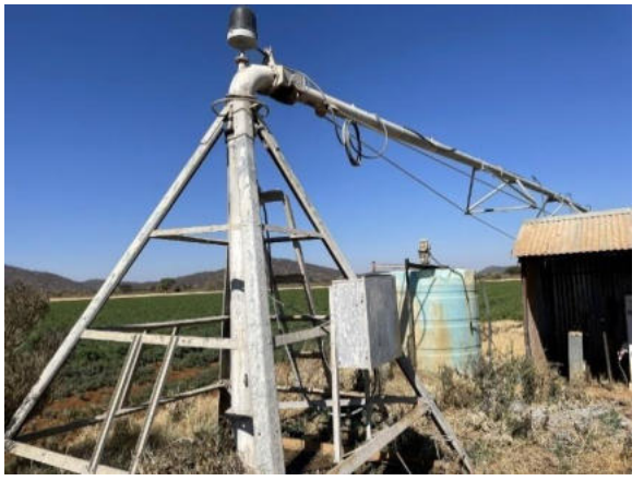
Photo 4-36 Typical centre pivot base
