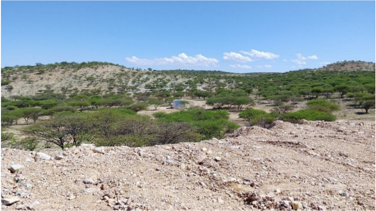
Image 3: Corrugated zinc structure on site
