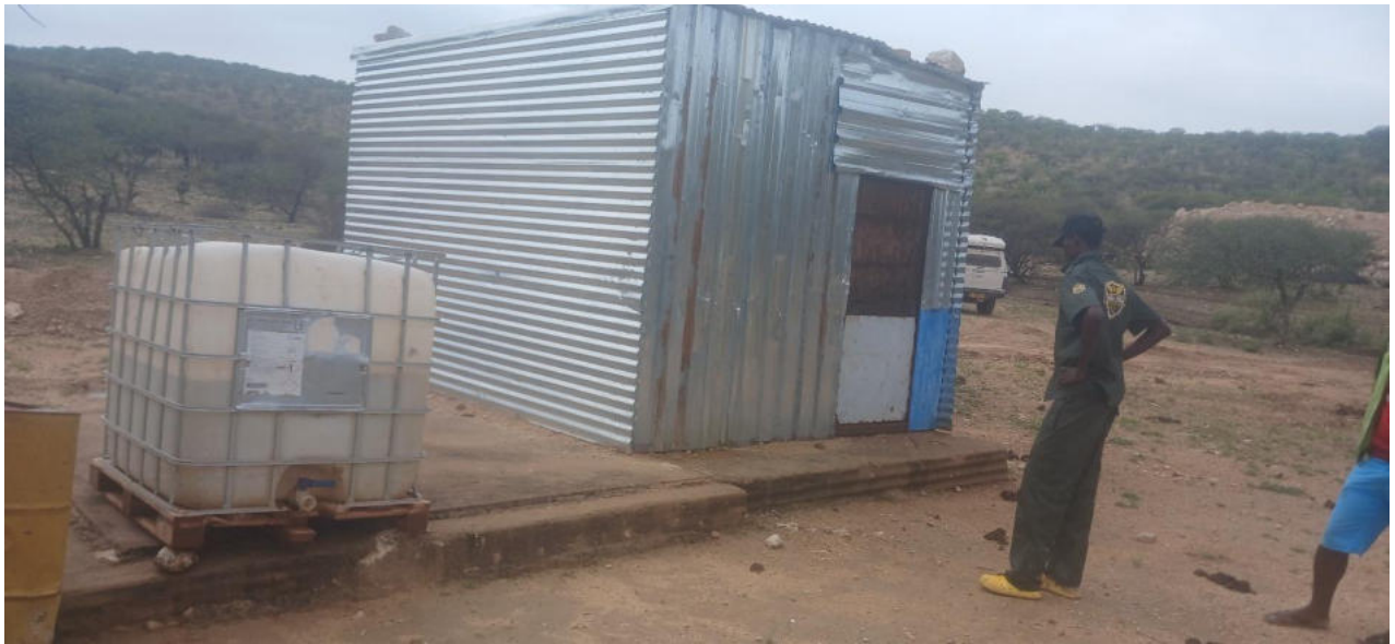
Figure 5: Water facility and security house with water tank at the gate hosting within mining claim 70310.
