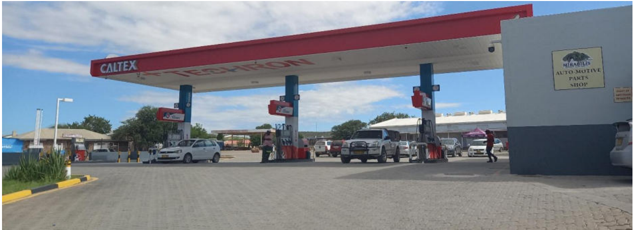
Figure 3: FRO seen from South to North
