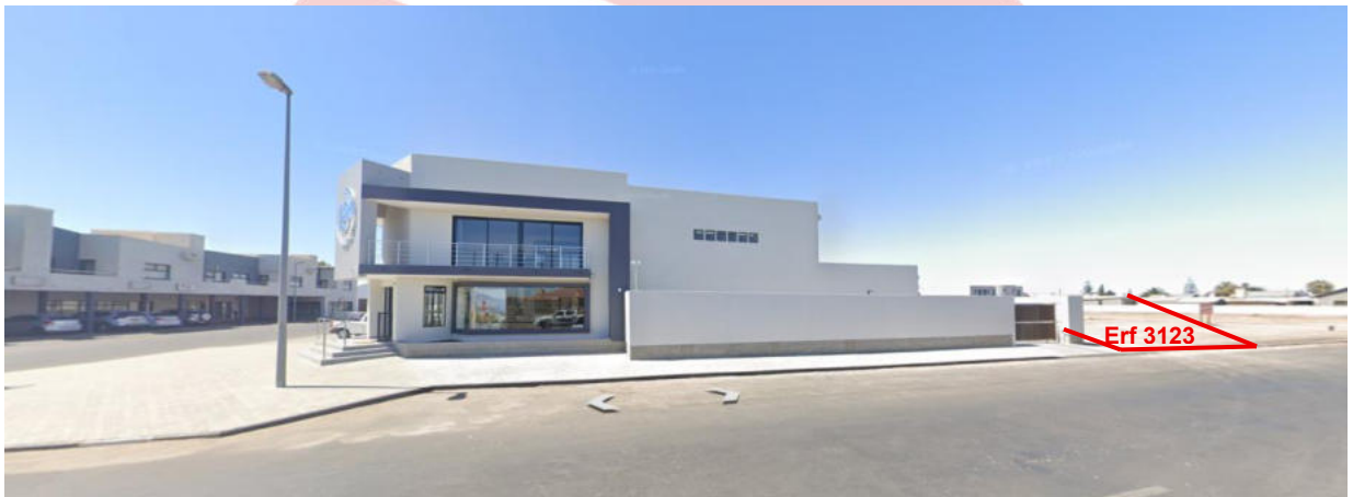
Figure 2: Side view of current Radio Electronics building.(Source: Google Earth, March 2024).
