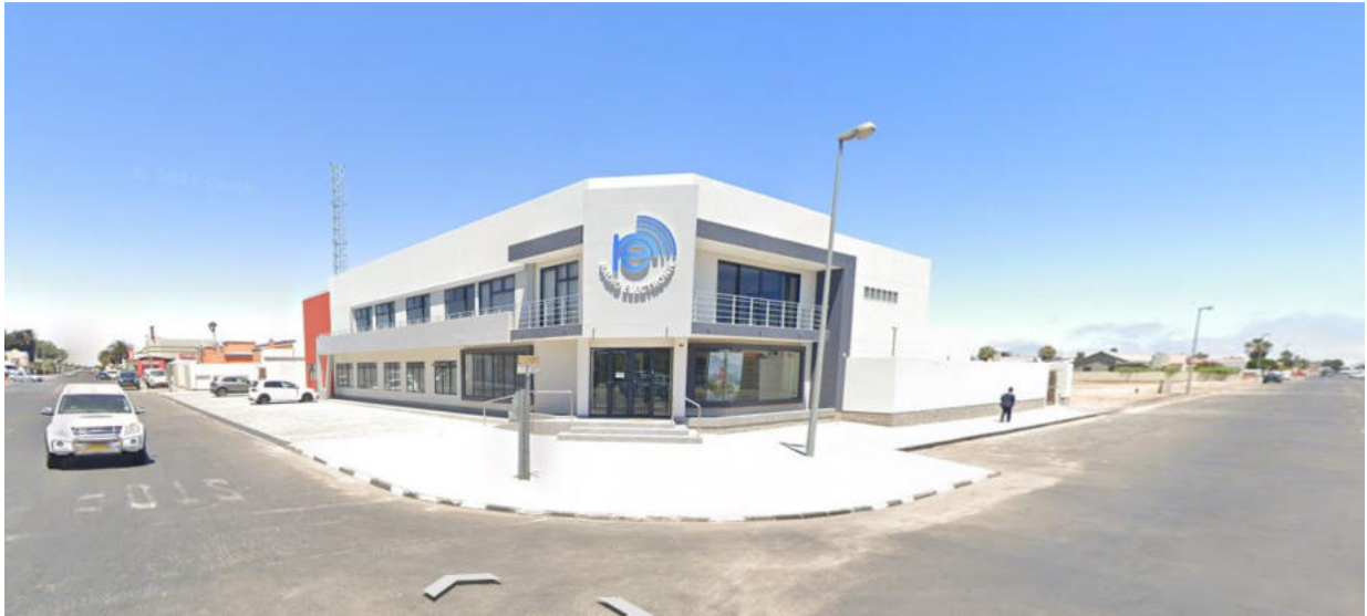
Figure 1: Front view of current Radio Electronic building (Source: Google Earth, March 2024).
