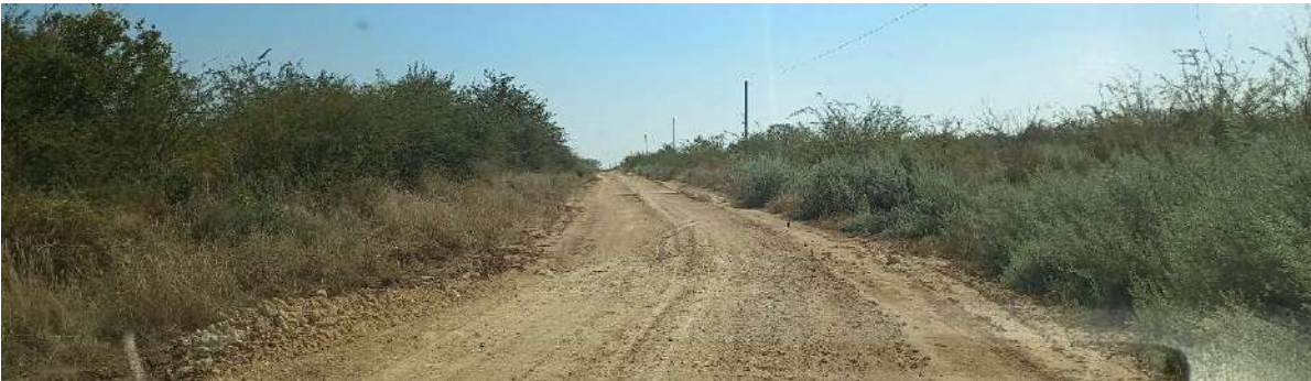
Figure 4: Access road to the borrow pit
