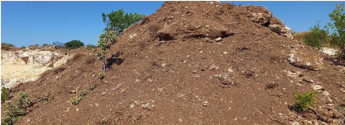
Figure 9: Topsoil stockpiled for rehabilitation
