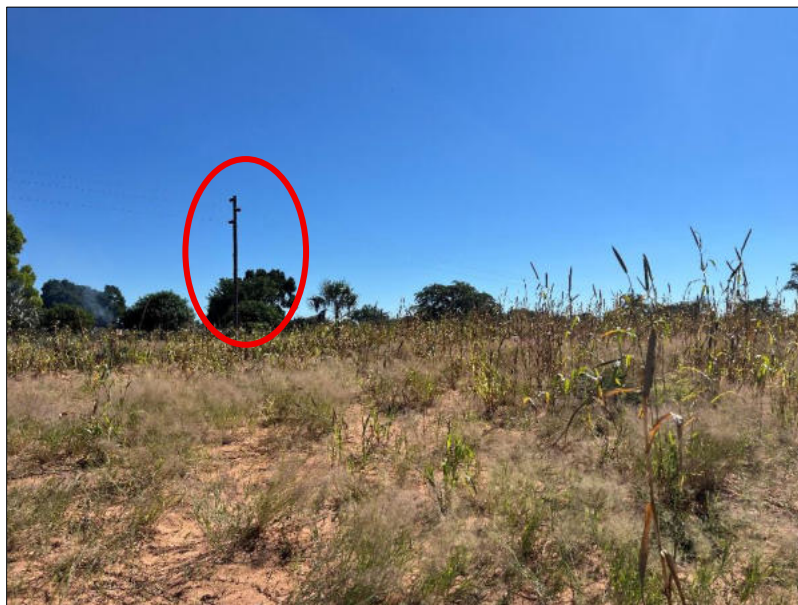
Figure 5-7: The nearest NORED power line to the western side of the site in Nkurenkuru Town
