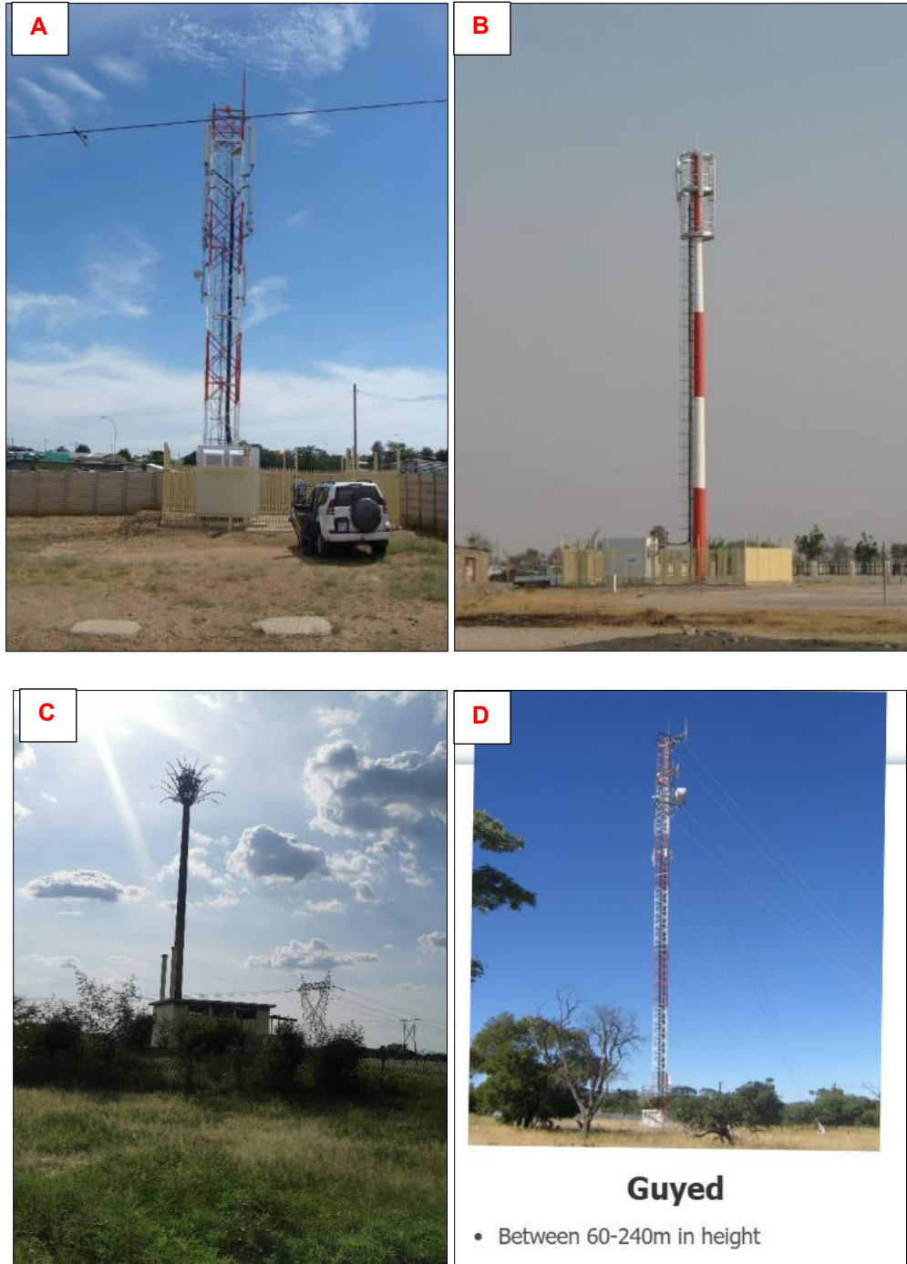
Figure 3-1: Types of network structures: A - Lattice, B - Monopole, C - Camouflage, and D – Guyed
