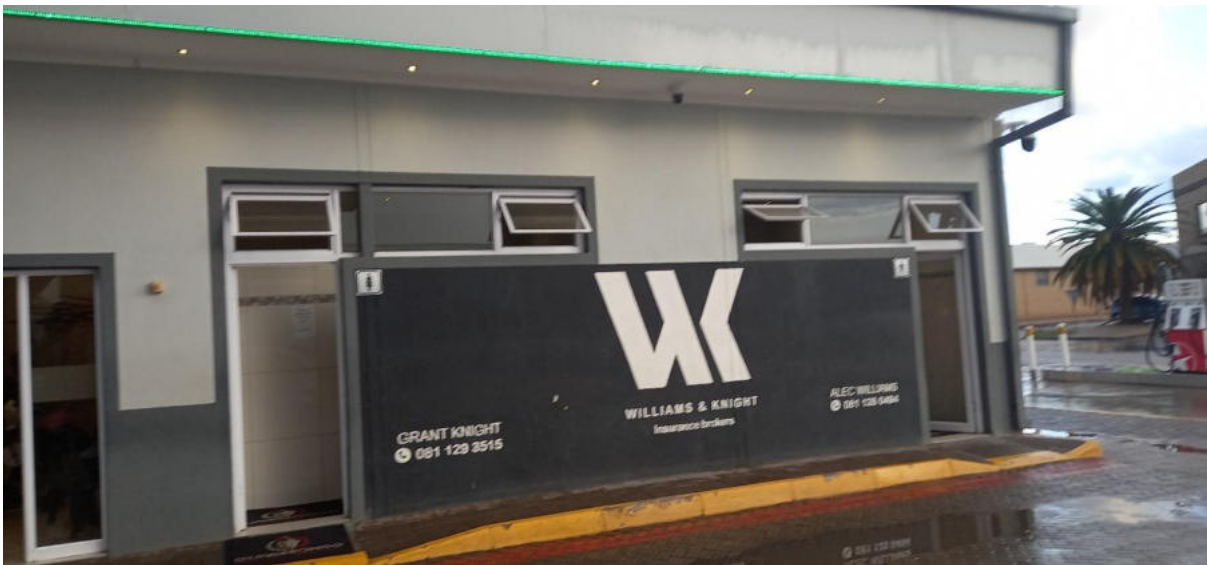
Figure 15: Toilet facilities at Caltex
