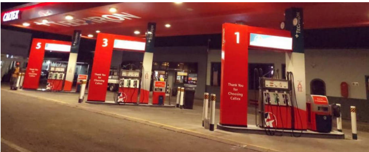
Figure 4: The canopied section of the fuel service station
