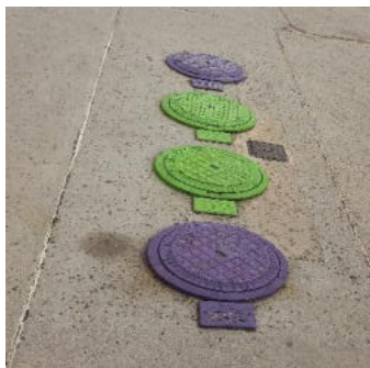
Figure 6: Colour coded USTs
