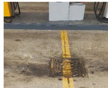
Figure 11: Forecourt runoff water drainage channel
