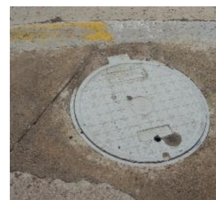
Figure 14: Paratus fibre-optic network manhole cover
