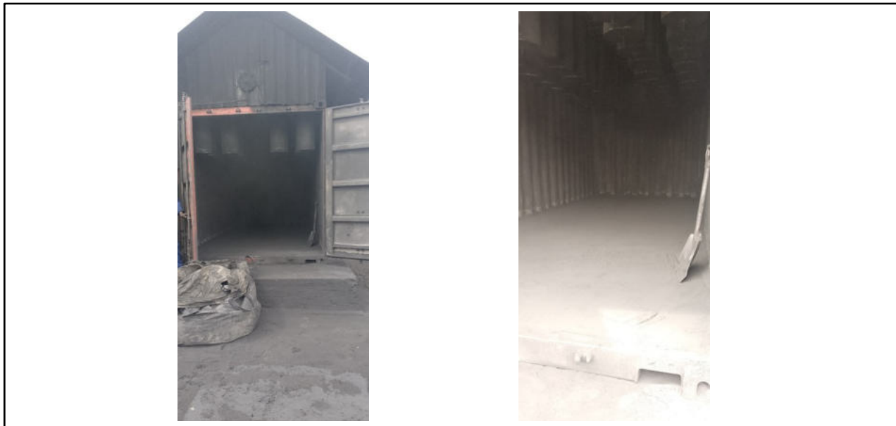
d) One of the dust collectors on site which is well cleaned
