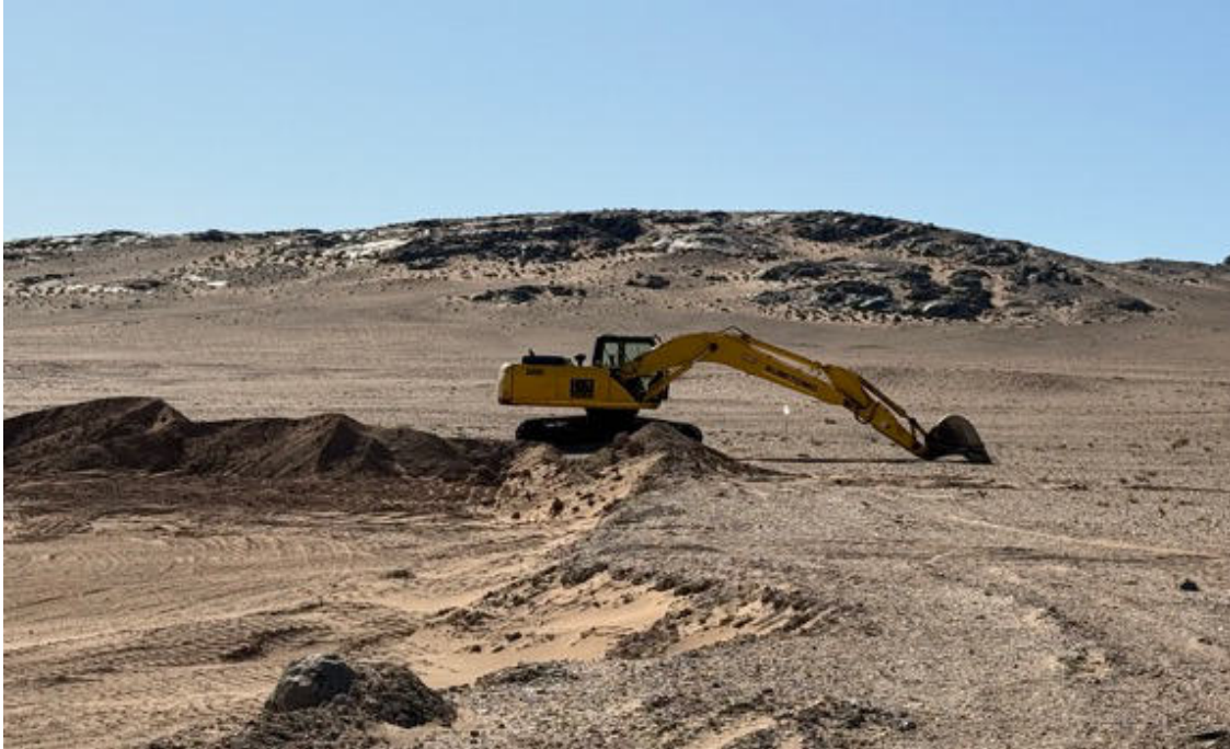
Figure 2-1: Current Gravel Mining Activities – Luderitz Town Council
