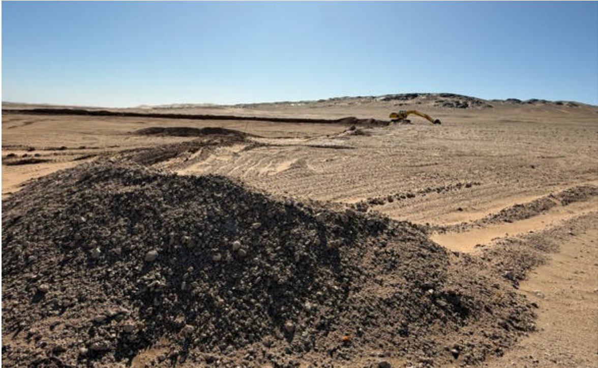
(Current Gravel Mining Activities by Lüderitz Town Council, 2025)
