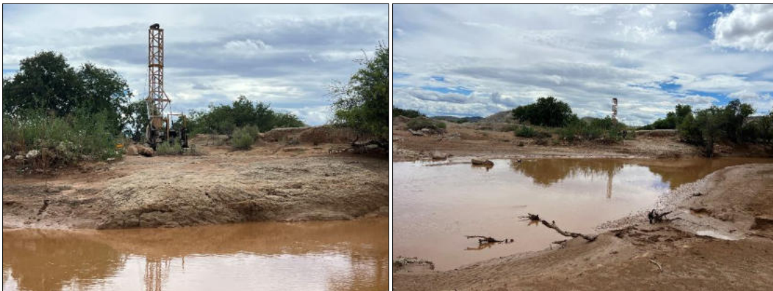
Figure 2-2: The ongoing project’s geotechnical investigation (geotechnical drilling) in March 2026
