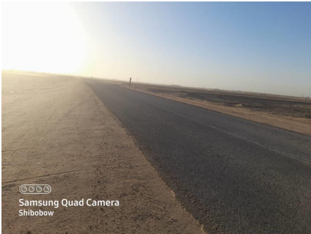
Figure 3: C14 Access-road to the project site
