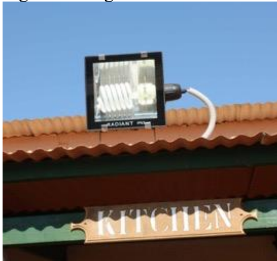
Figure 12: Light Fixture Removed
