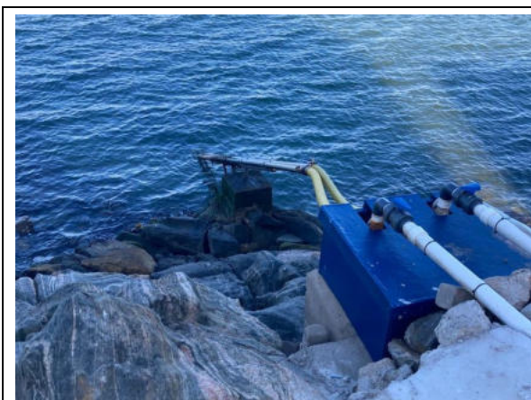
Photo 4-11 Seawater abstraction point
