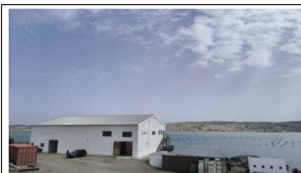
Photo 4-5 Processing plant from the outside
