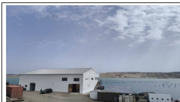
Photo 4-5 Processing plant from the outside
