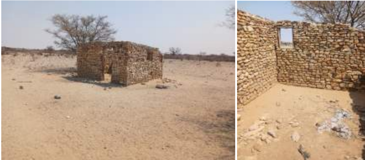
Figure 28 - The ruined stone-built structure on farm Aniswept (Source: Nankela, 2025)
