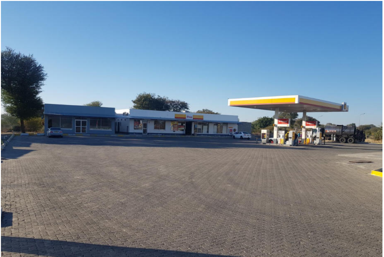
Photo 1. The existing Bukalo Service Centre .
