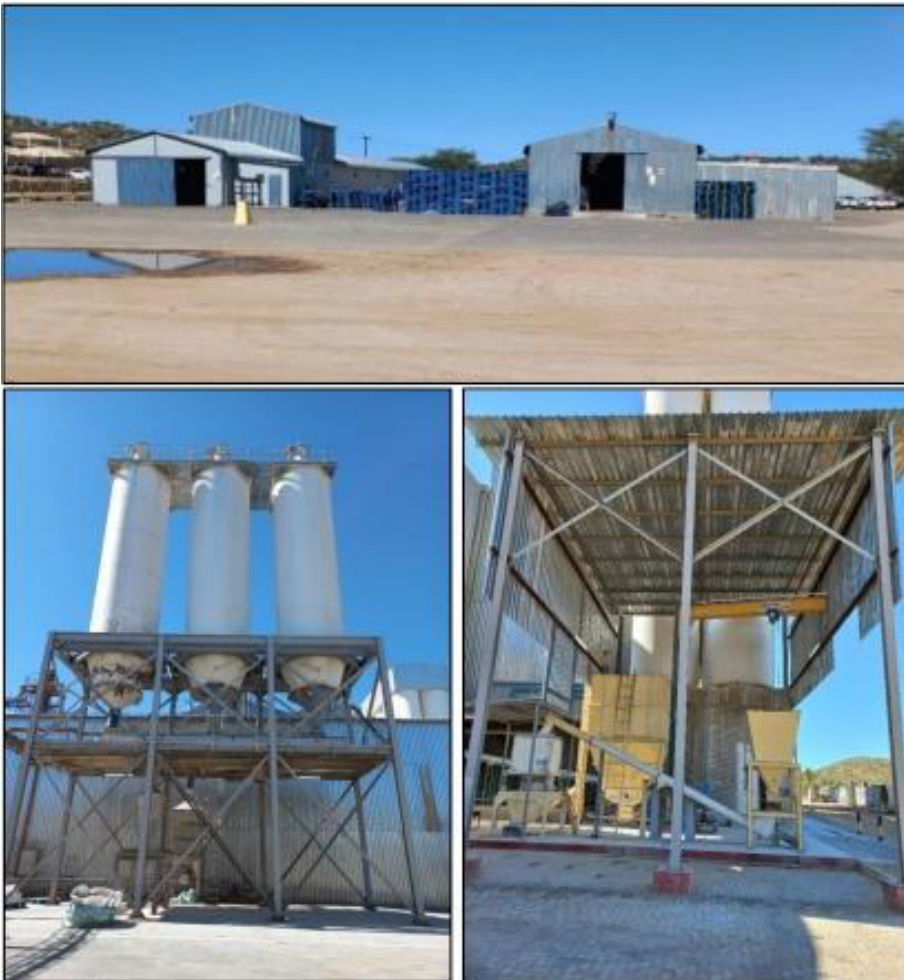
Figure 5 : Warehouse stores and silos
