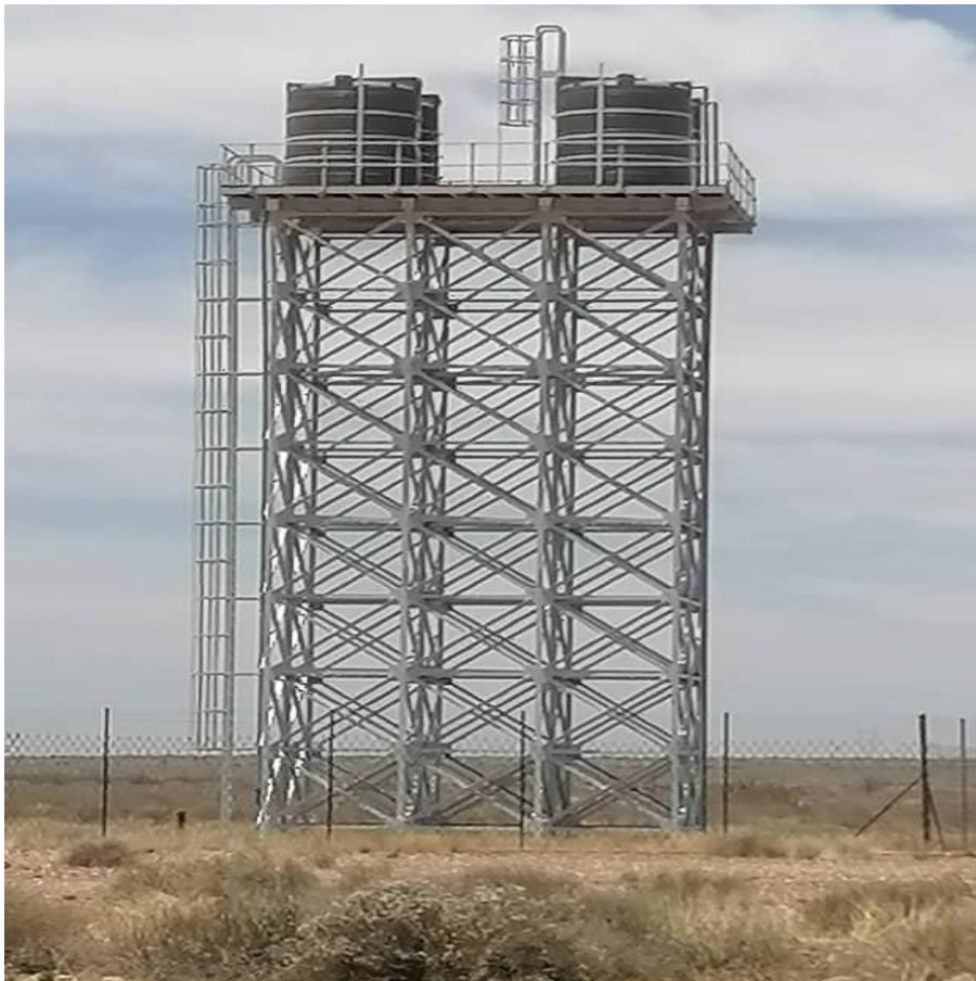
Figure 7: Water Reservoir and the Water Tower west of the proposed site location
