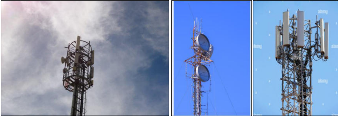
Figure 2-2: Different types of panel-type antennae
