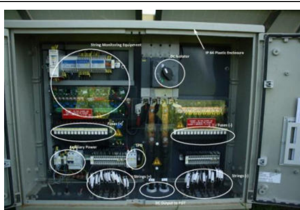
Photo 5-4 Typical enclosure components
