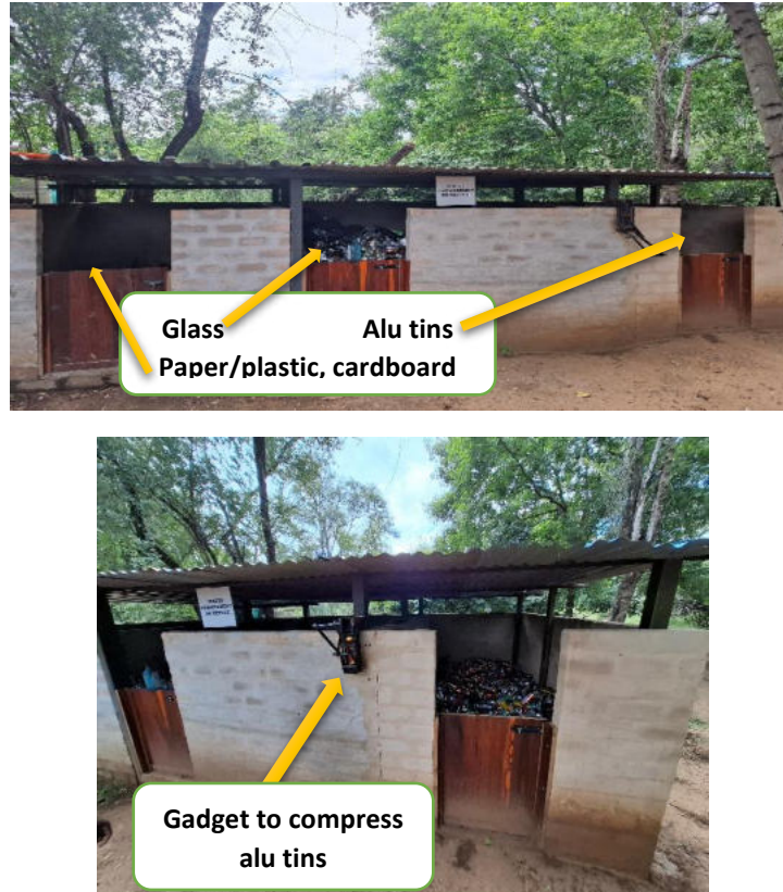
Figure 9: Cubicles for storage of solid waste prior dispatch for recycling
