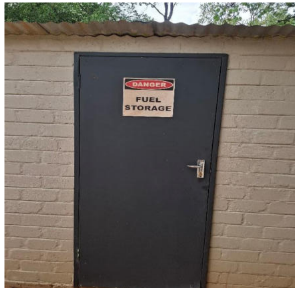
Figure 23: Secure storage for fuel.
