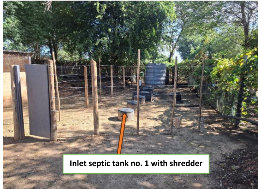
Figure 15: Stage 2: The 7-tank digester system in place with purified water stored in the 5000-liter tank for the compost and fruit trees
