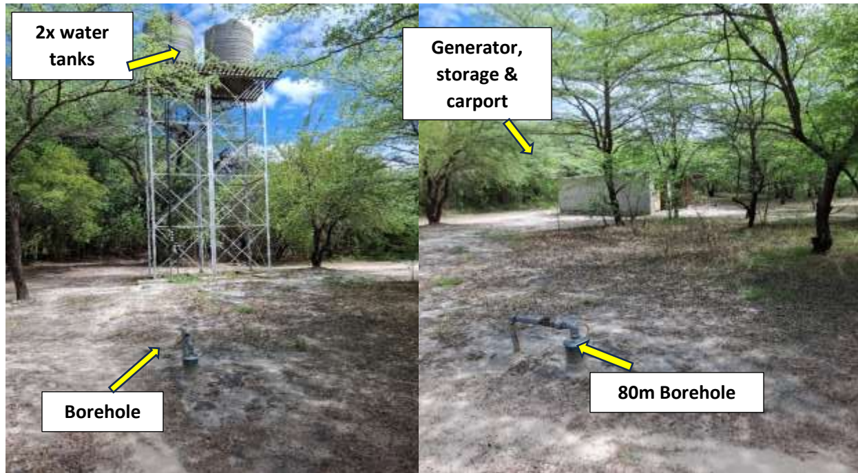
Figure 7: The borehole at 80m depth and a capacity of 2 cubic meter (m 3 ) per hour with 2x 5000-liter tanks (LHS) and carport & generator in the background (RHS) (E Klingelhoefter).
