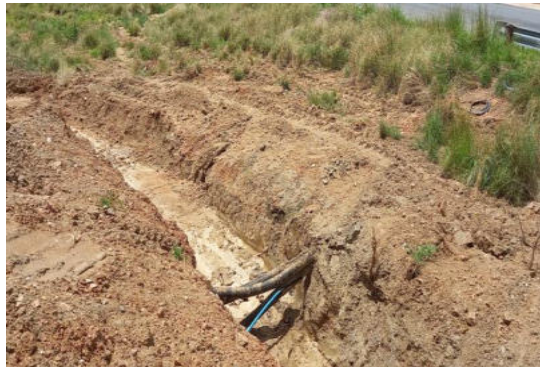
Figure 10: Exposed Electrical Cables at the Project Site
