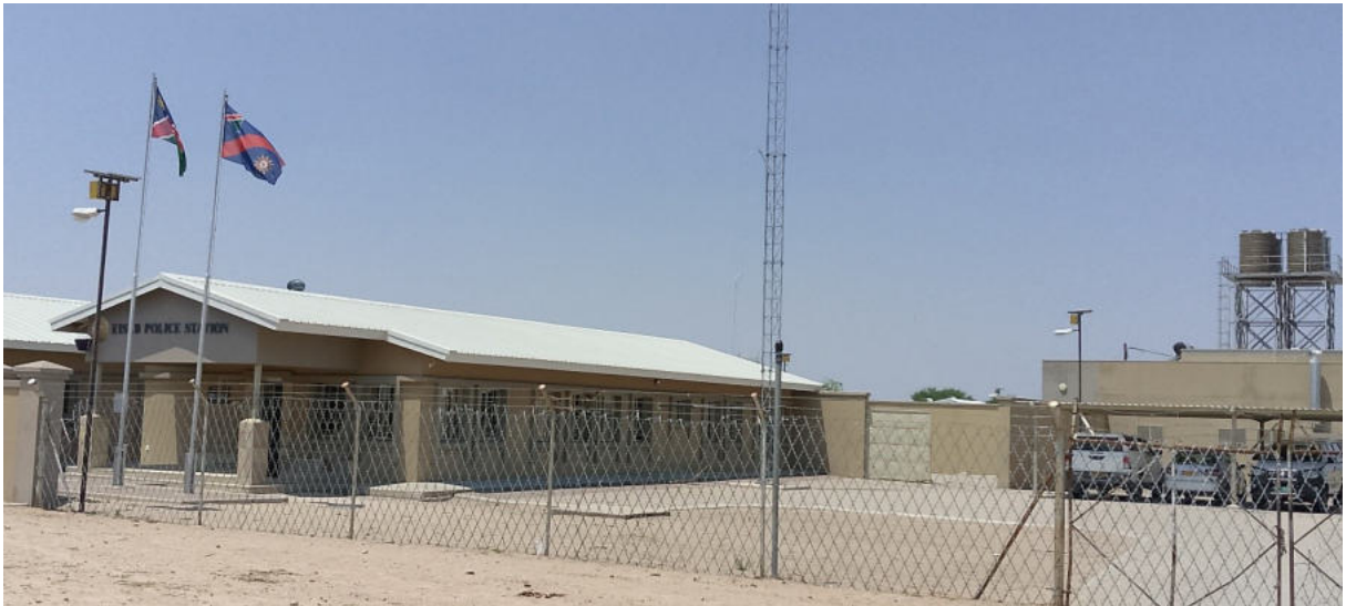
Site image 1: : Eiseb Police Station
