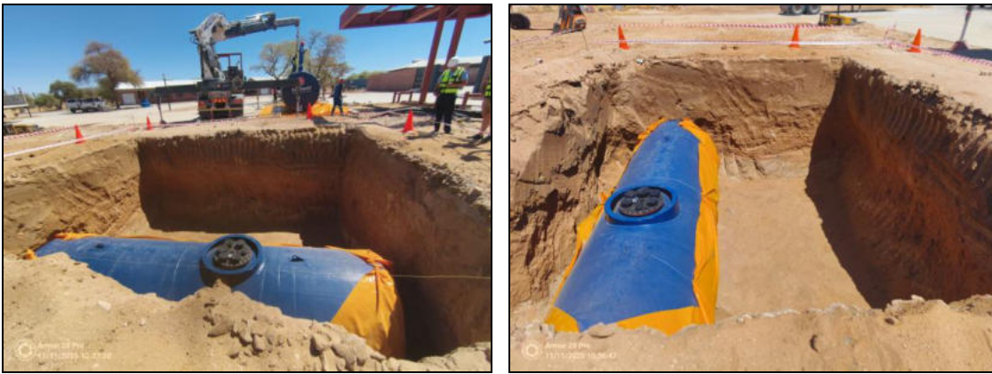
Figure 6: During the construction of the facility
