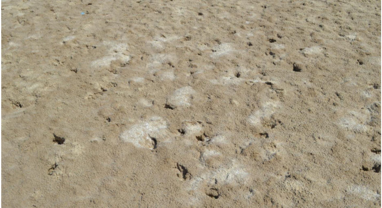
Figure 18: Soft and unstable ground
