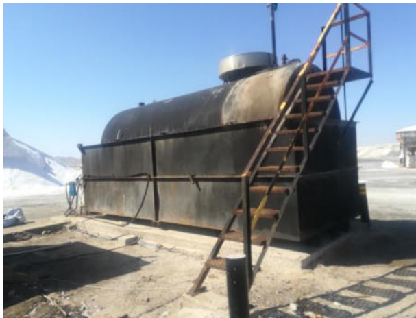
Photo 1. Existing 23m 3 tank in containment structure
