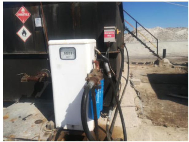
Photo 2. Dispenser on concrete containment floor
