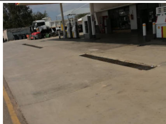
Photo 4-3 Drains to oil-water separator
