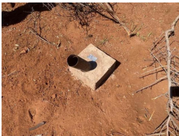
Photo 4-9 Example of a borehole ((Votorantim site)
