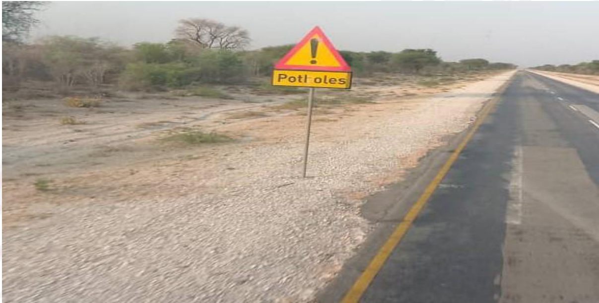
Picture warning motorist of potholes.
