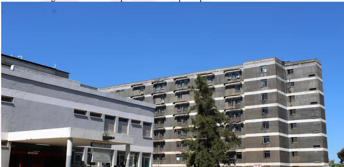
Ndola teaching hospital along Kabwe road
