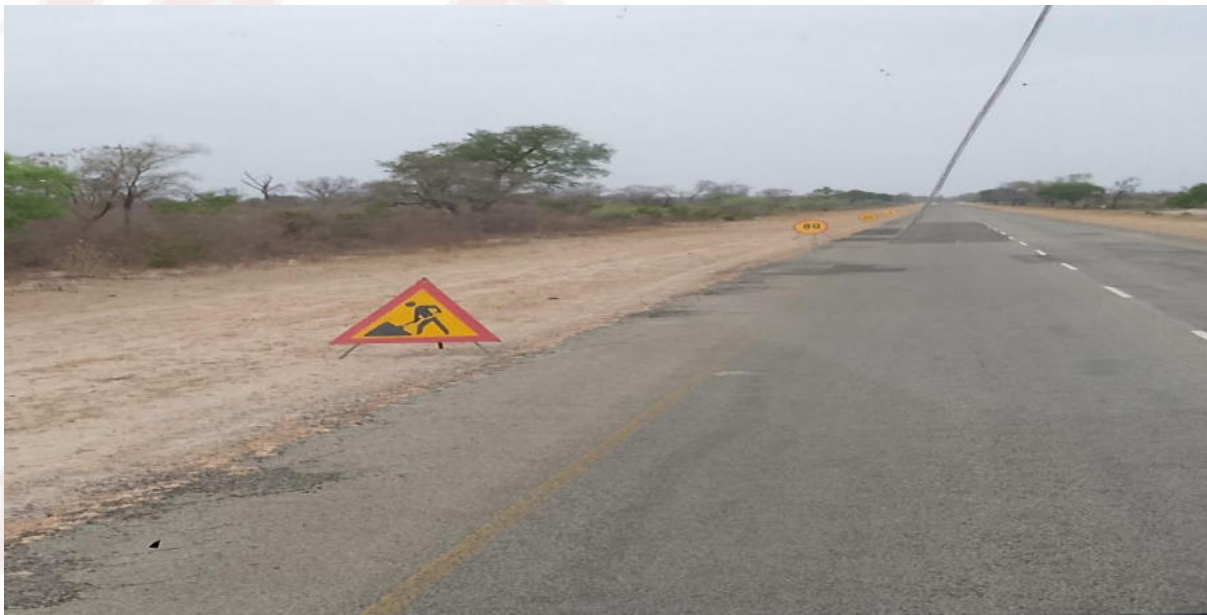
Pothole Patching along the B8 road as you head to Kongola
