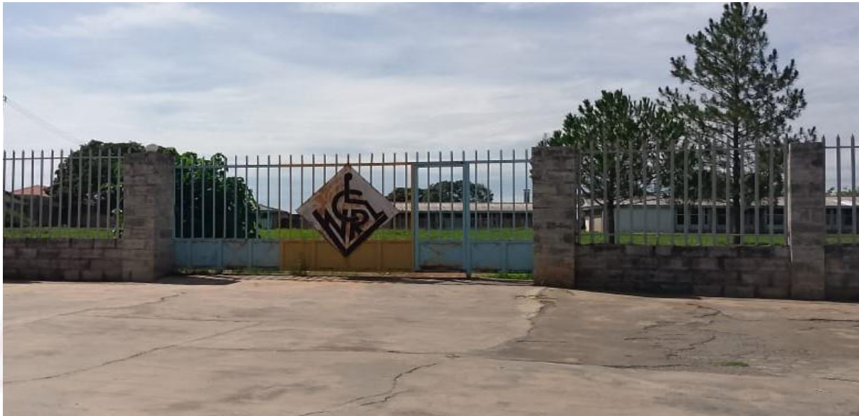
Picture showing training center for people living with disability along Ndola-kitwe dual carriageway
