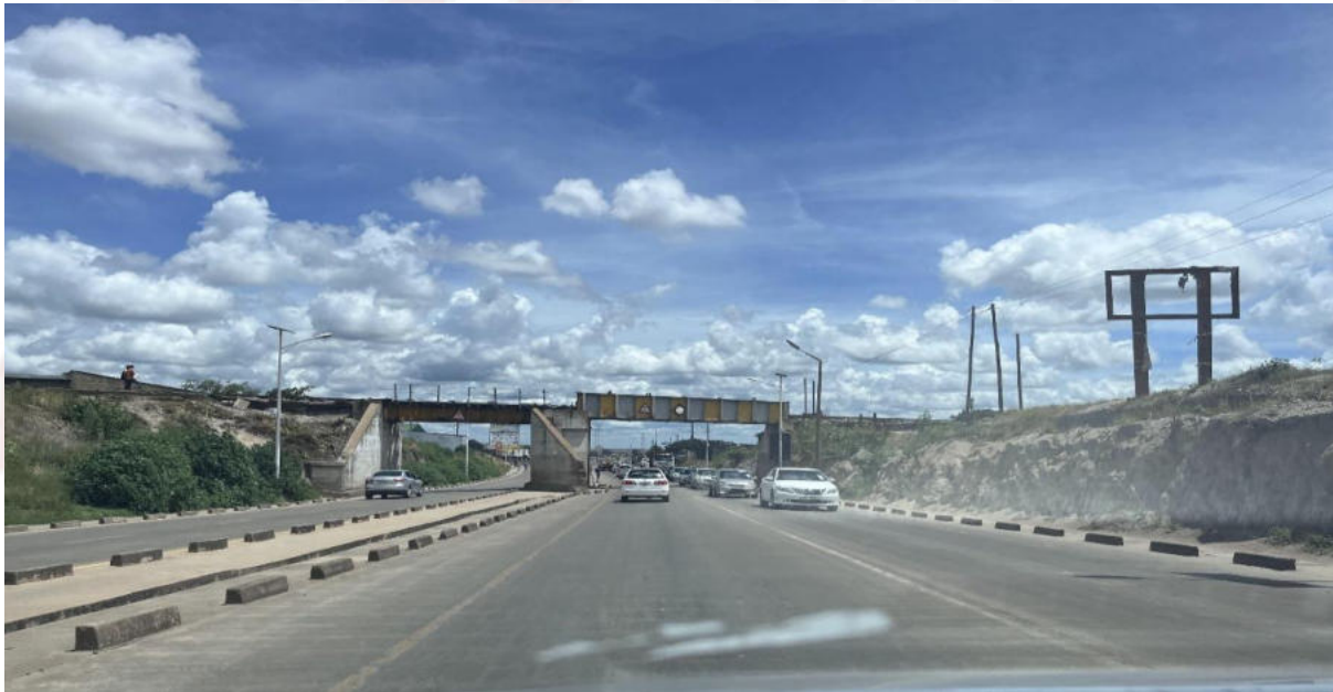
Fly over bridge with height limit of 4.8 metres as you leave Chingola
