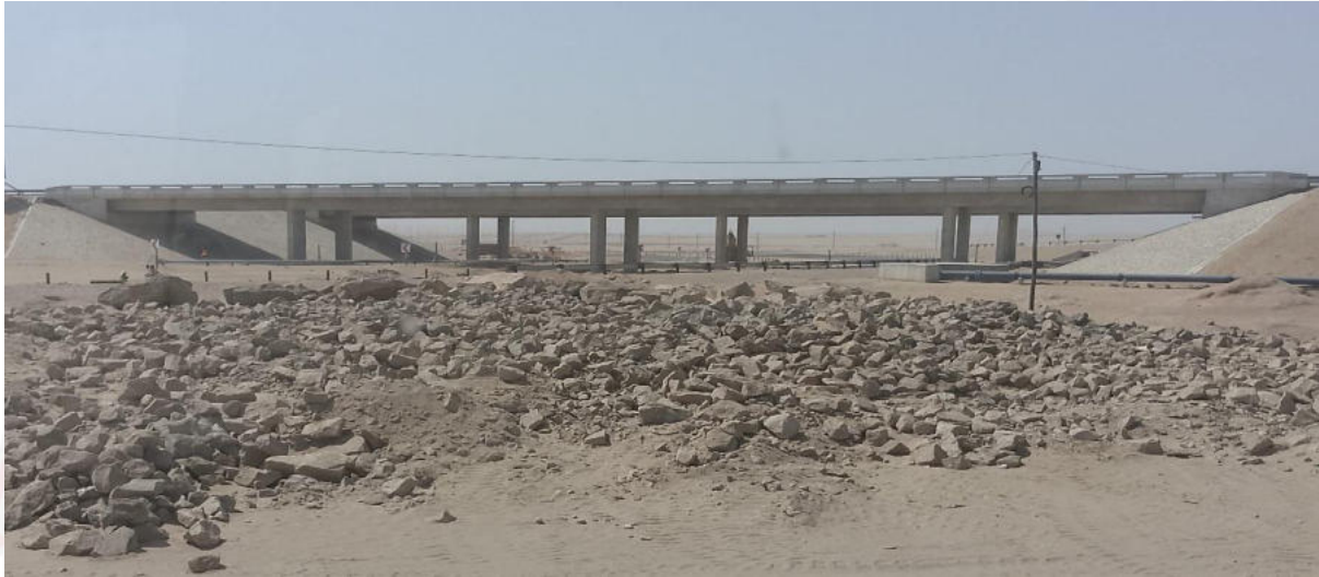
The Dune 7 Bridge under construction
