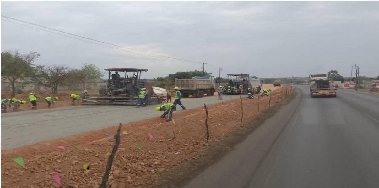
Ndola-Lusaka dual carriage way under construction
