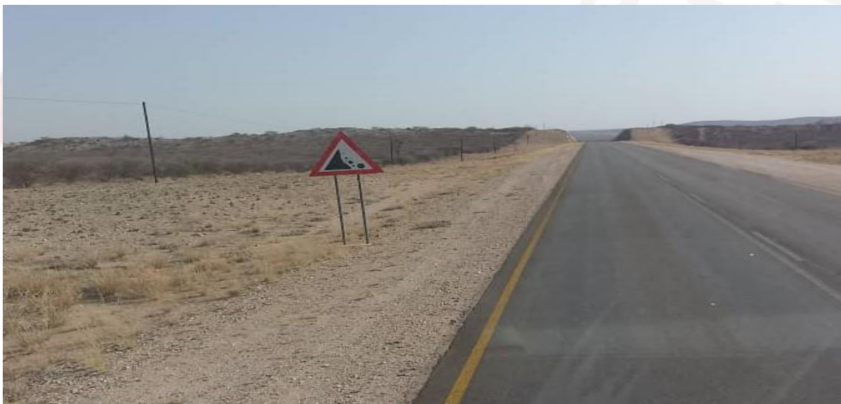
Picture showing rocks falling as road cuts between a mountain.
