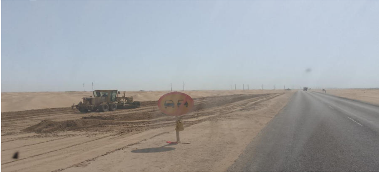
A new road under construction
