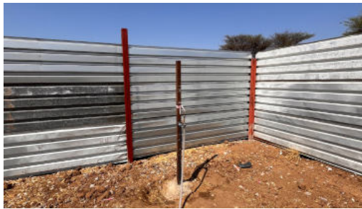
Water Tap on site
