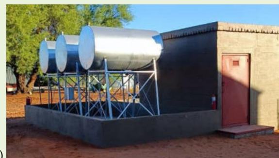
Figure 3: Pictures showing: a) the three (3), 2,200-litre diesel storage tanks at Farm Hartebeestloop No. 202 (Source: L Maartens, 06 June 2022); and b) the completed bunded enclosure (December 2023) (Source: Tristone Business Trust, 07 August 2023).
