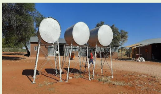
Figure 3: Pictures showing: a) the three (3), 2,200-litre diesel storage tanks at Farm Hartebeestloop No. 202 (Source: L Maartens, 06 June 2022); and b) the completed bunded enclosure (December 2023) (Source: Tristone Business Trust, 07 August 2023).
