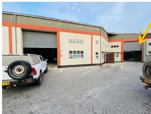
Figure 1 –Image showing existing warehouse
