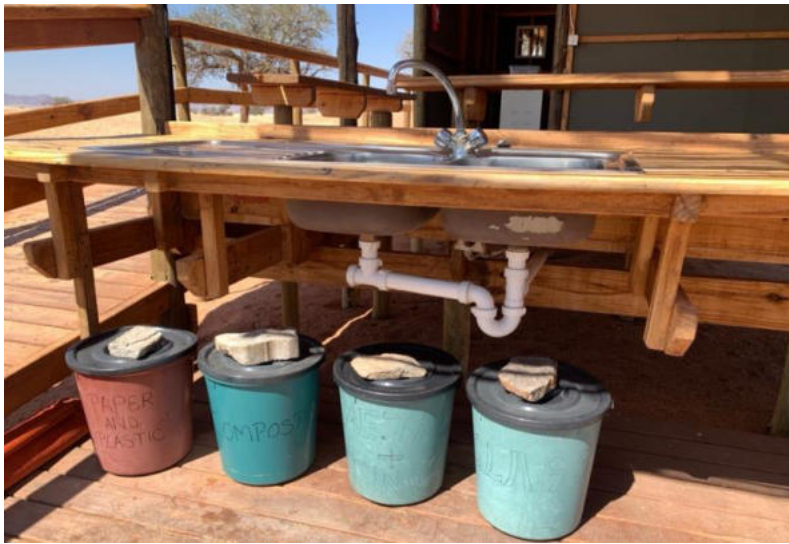
Figure 12. Lidded rubbish bins under the food preparation counter.
