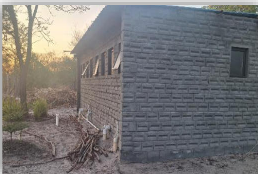
Behind the Public Sanitary Rooms
