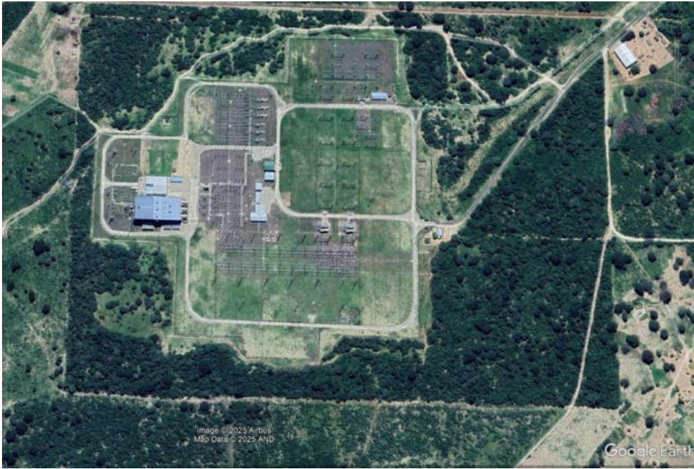
Figure 9: Existing Nam-Power Electrical Grid next to the Solar power plant
