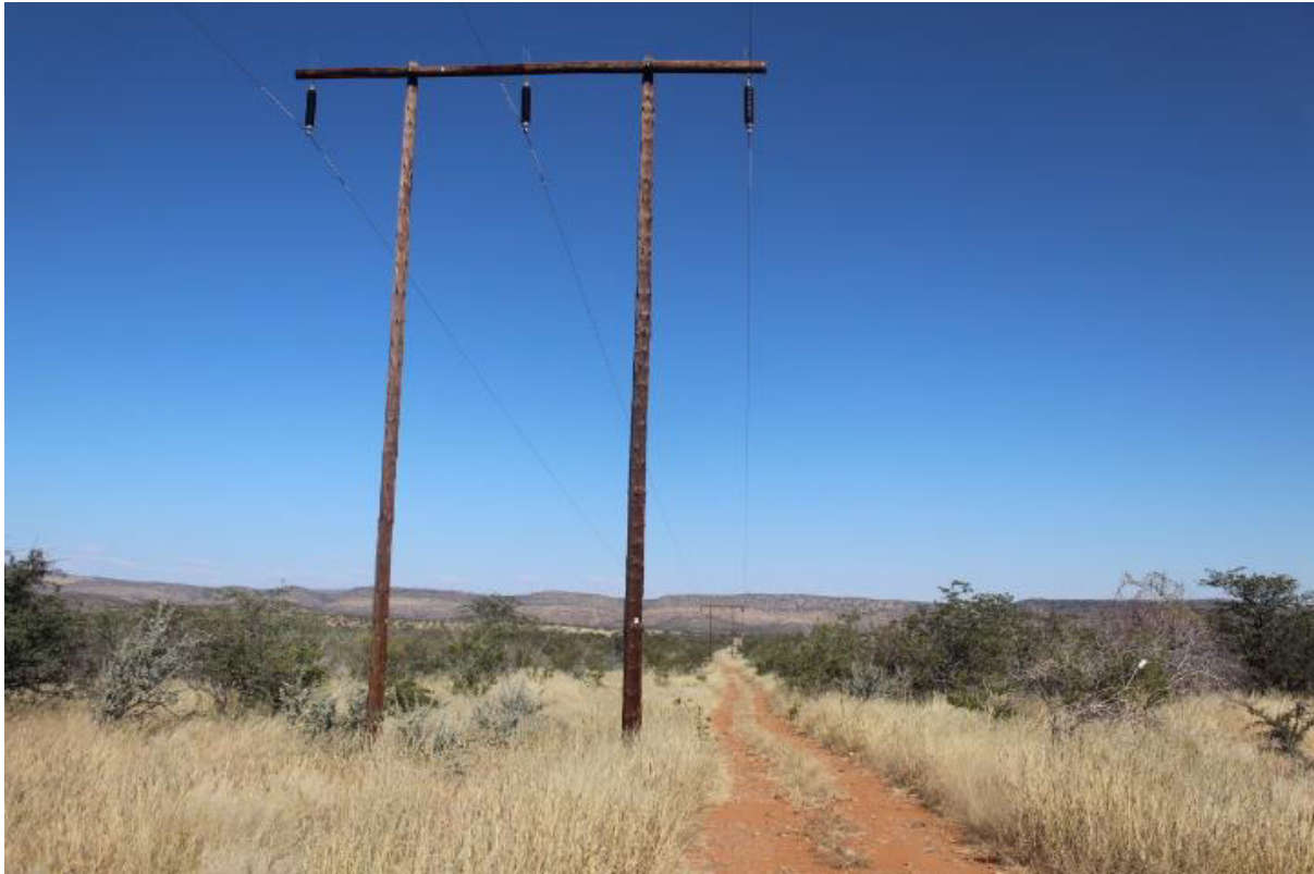
Figure 4: Existing road (track) in the area that will be used to access the mining site.
