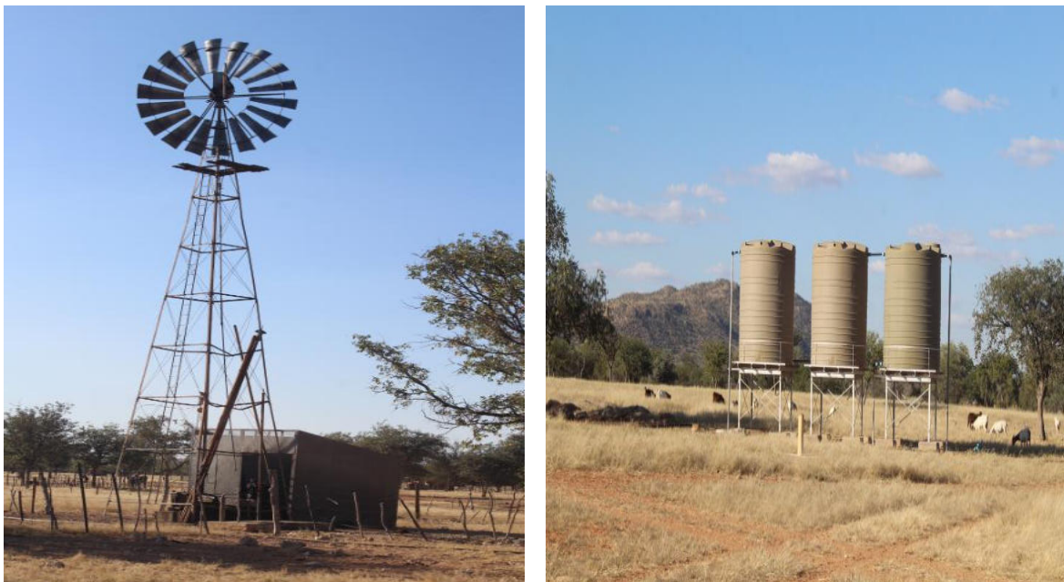
Figure 3: Existing water infrastructures in the area.
