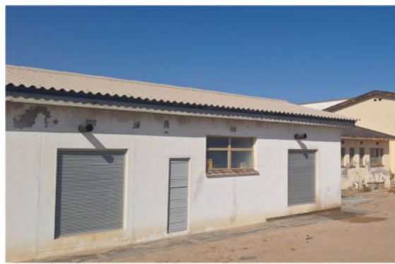
Photo 3-11 Backup generator room with small diesel spill
