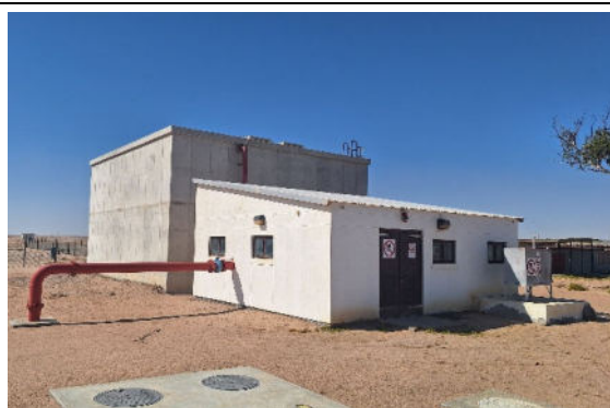
Photo 3-9 Water reservoir and pump room
