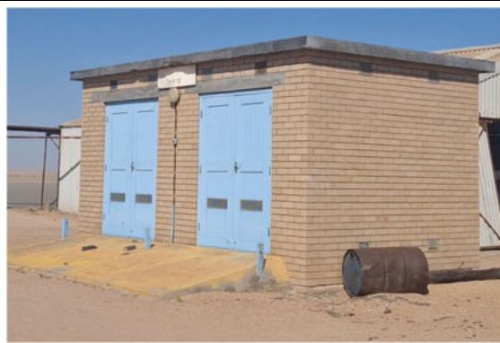
Photo 3-15 Emergency chemical storage
