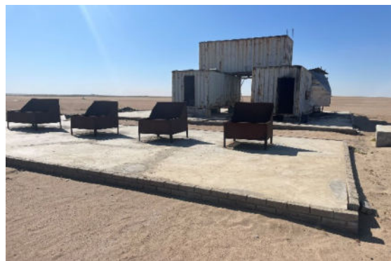
Photo 3-3 Firefighting training area
