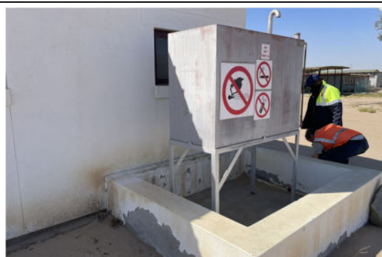
Photo 3-10 Water pump fuel storage
